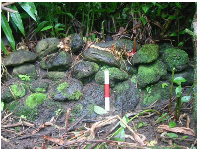
Figure 6. Section of wall that divides terraces 272-c and 272-e, facing south. The scale is marked in 10 cm increments.
